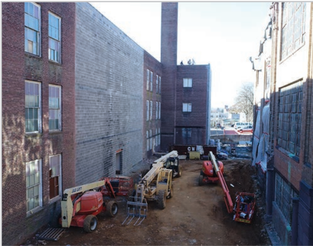
Walls being rebuilt where connecting hallways previously existed.
