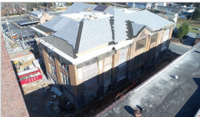
New roof being installed.
